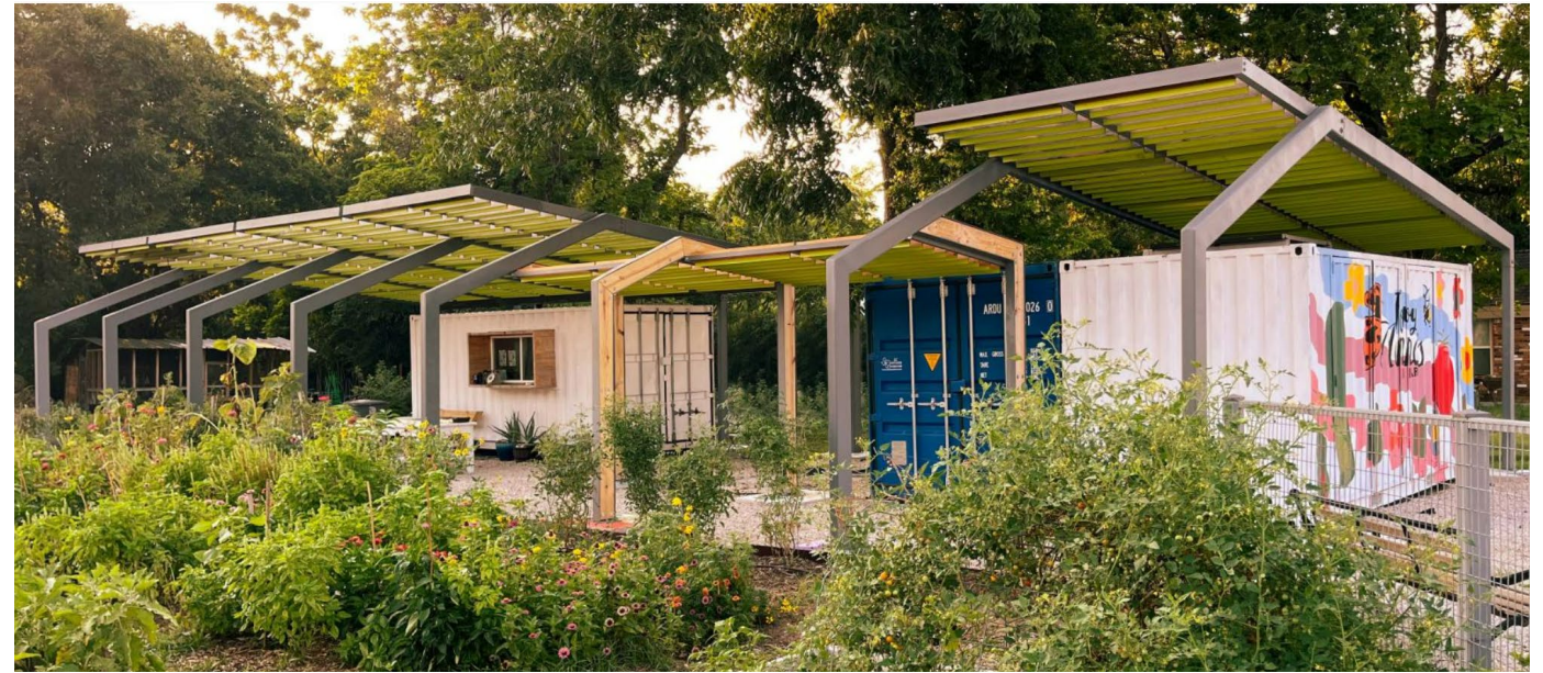
PAVILION IN USE
